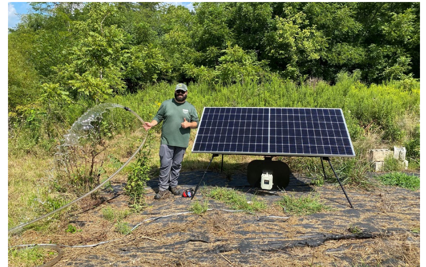
Cincinnati Nature Center Native Plant Manager Jake Sberna poses with the solar-powered water pumping system.
