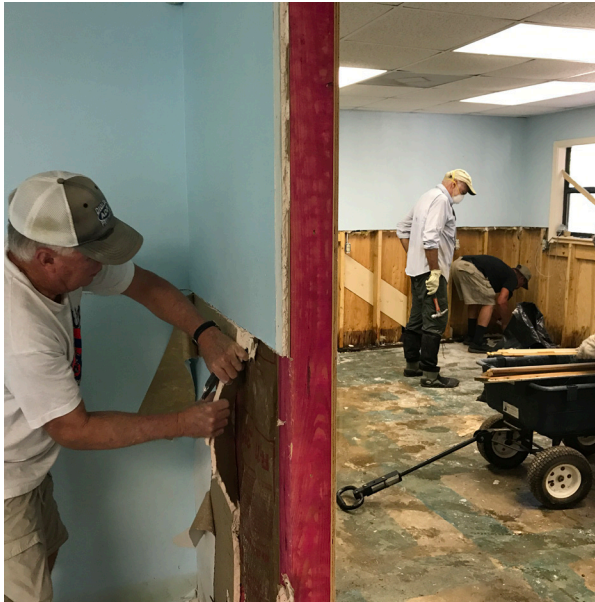
Gulf Coast Bird Observatory staff and volunteers gutting the field house
