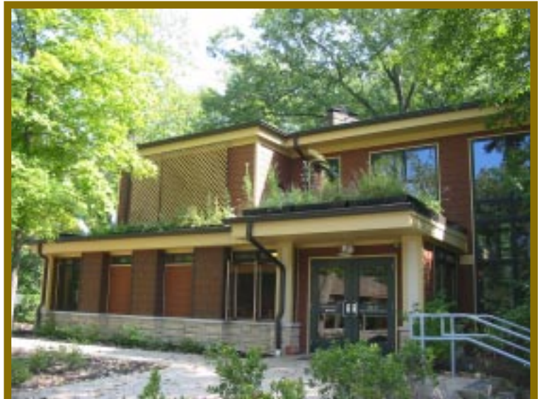
photo by Nature Center at Shaker Lakes
